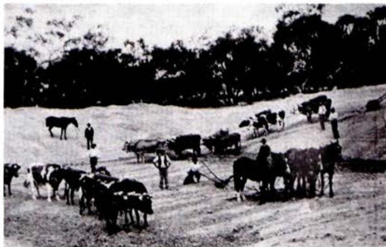
Tank-sinking near Birchip, using bullocks and horses.
