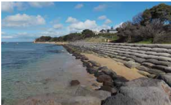
Temporary sandbag seawall at Portsea front beach, to be replaced by a rock revetment. Photo: R Molloy
