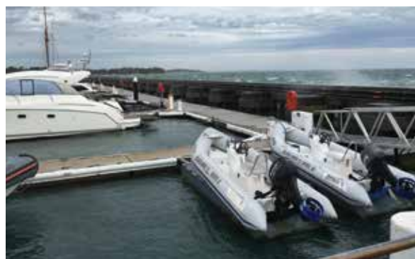
Blairgowrie Yacht Squadron Marina includes components to enhance biodiversity and reduce its ecological impact – these include a wave attenuator instead of a breakwater, and relocation and attachment of sponges and ascidians to the marina's planking. Photo: R Molloy
