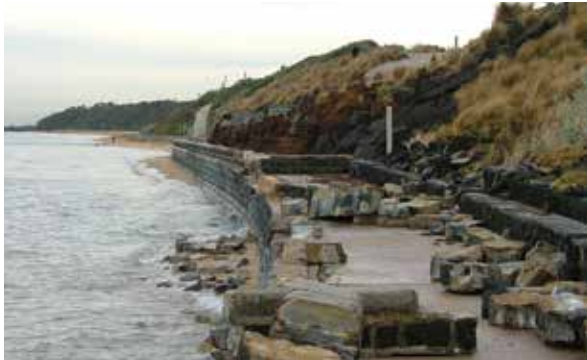
Bluestone masonry seawall at Black Rock, constructed in the 1930s, has sustained significant storm damage. A rock revetment along the existing seawall is to be built to protect the historical bluestone seawall, promenade and adjacent cliffs from erosion. Photo: M Mitchell
